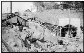
The Newcastle tunnel is under construction in 1909. The tunnel will house the new second track as well as the realigned original track which can be seen at lower left. See pp. 2 &4 for more details
