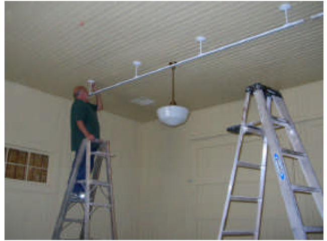
TONY HESCH PUTTING FINISHING TOUCHES ON MUSEUM TRACK LIGHTING.
