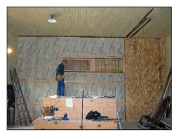
In the photos above, the north wall of the baggage room required the addition of a section of plywood sheer wall to meet earthquake standards. The beaded tongue-and-groove boards were removed from the entire wall and insulation added along with shear plywood at far right corner and nailing strips.
