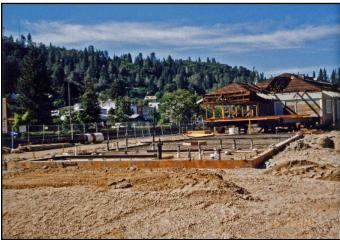
The depot building was lifted off its old foundation and moved a few hundred feet toward Grass Valley St. A new foundation was poured at the old site with utility stub-outs. The building was then moved back in place and bolted to the new foundation. Note the hole in the roof for inserting the glue-laminate beam.
