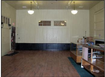
Above left, original boards were reinstalled along with custom-milled replacements. After the room was painted, simulated oak flooring was installed to complete the look. In the photo at right note the operational sliding door at far left next to the new doorway being installed, and simulated wainscot to cover boards cut off above the foundation attachments and new electrical wiring.
